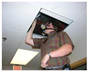
Figure 1. PMPs may be exposed to environmental risks on the job. The man is wearing a respirator but should also be wearing gloves when inspecting drop ceilings. Photo by Erin Bauer.
