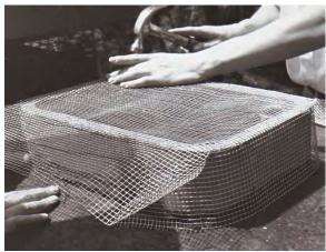
Figure 9. Never use hardware cloth to secure a chimney, as shown in photo. Use professionally manufactured chimney caps. Photo by Stephen M. Vantassel.
