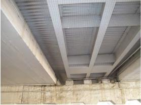
Figure 5. A net has been suspended below this bridge to prevent birds from nesting on the I-beams. Photo by Stephen M. Vantassel.
