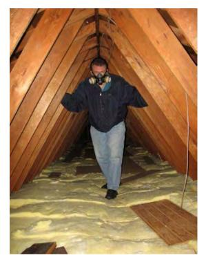
Figure 8. Hold rafters while probing for floorboards. Feel for joists with your feet or hands, or pull back the insulation to locate them. Photo by Stephen M. Vantassel.
