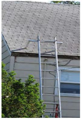
Figure 5. A stabilizer helps to keep a ladder away from a structure and increases stability. The electrical power line should be shut off before placing a ladder at a location such as this. Photo by Stephen M. Vantassel.
