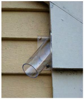
Figure 26. A BatCone<sup>™</sup> can be used as a one-way door to exclude birds. Photo by Jim Dreisacker.
