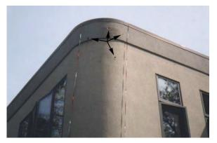
Figure 6. Arrows point to downy woodpecker holes in the synthetic stucco. The vertical lines are Mylar® tape installed when the damage began. Photo by Stephen M. Vantassel.
