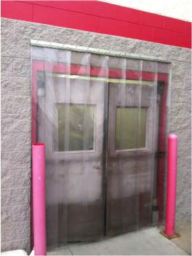
Figure 15. Plastic strips allow access by people and forklifts while preventing entry by birds. Photo by Stephen M. Vantassel.
