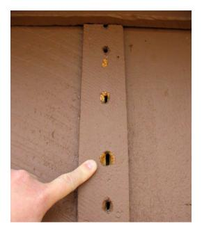
Figure 4. Damage to a building caused by woodpecker feeding. Photo by Stephen M. Vantassel.
